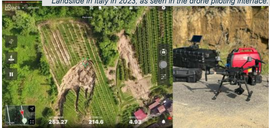
Landslide in Italy in 2023, as seen in the drone piloting interface.
