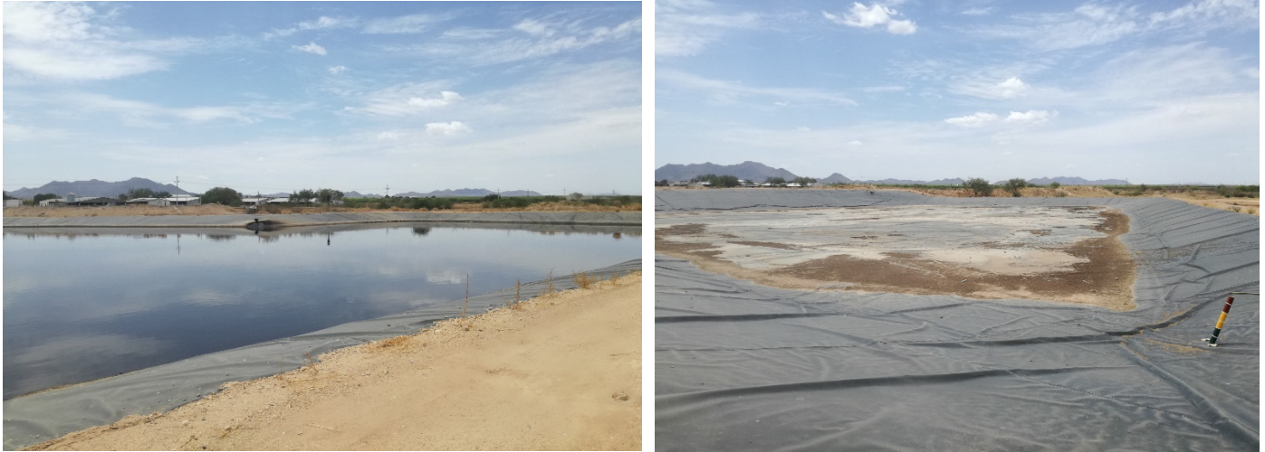
Figure 8. Evaporative ponds; no methane capture and use/burning no proper treatment and reuse of water and nutrients.
