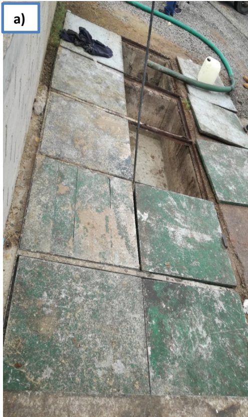
Figure 16. a) Fat trap and b) Manure waste channels at Pegson slaughterhouse.
