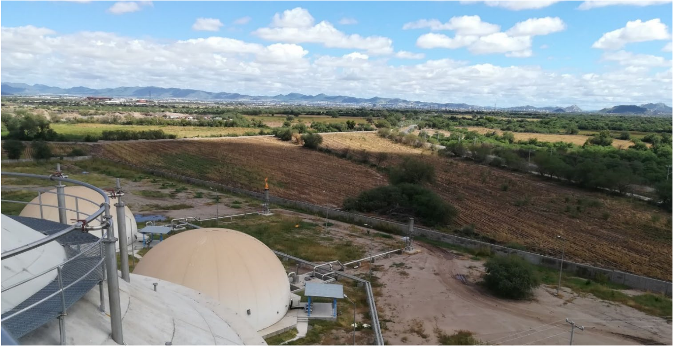
Figure 31. Roof on anaerobic digester, gasholders, biogas burners and agricultural lands nearby Hermosillo WWTP
