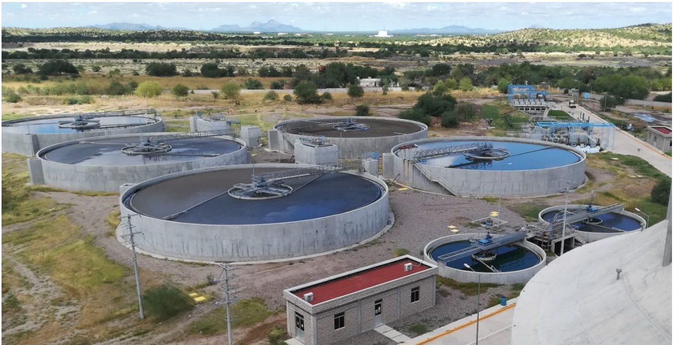
Figure 27. Pretreatment, primary settlers, gravity thickeners in Hermosillo WWTP
