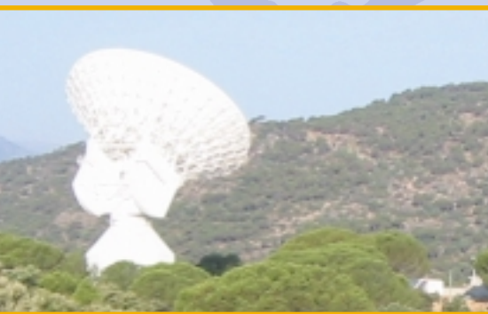
The ESA deep space antenna in Cebreros, Spain
