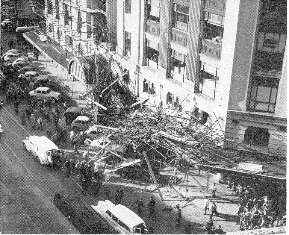
Earliest photograph taken of collapsed scaffold.
