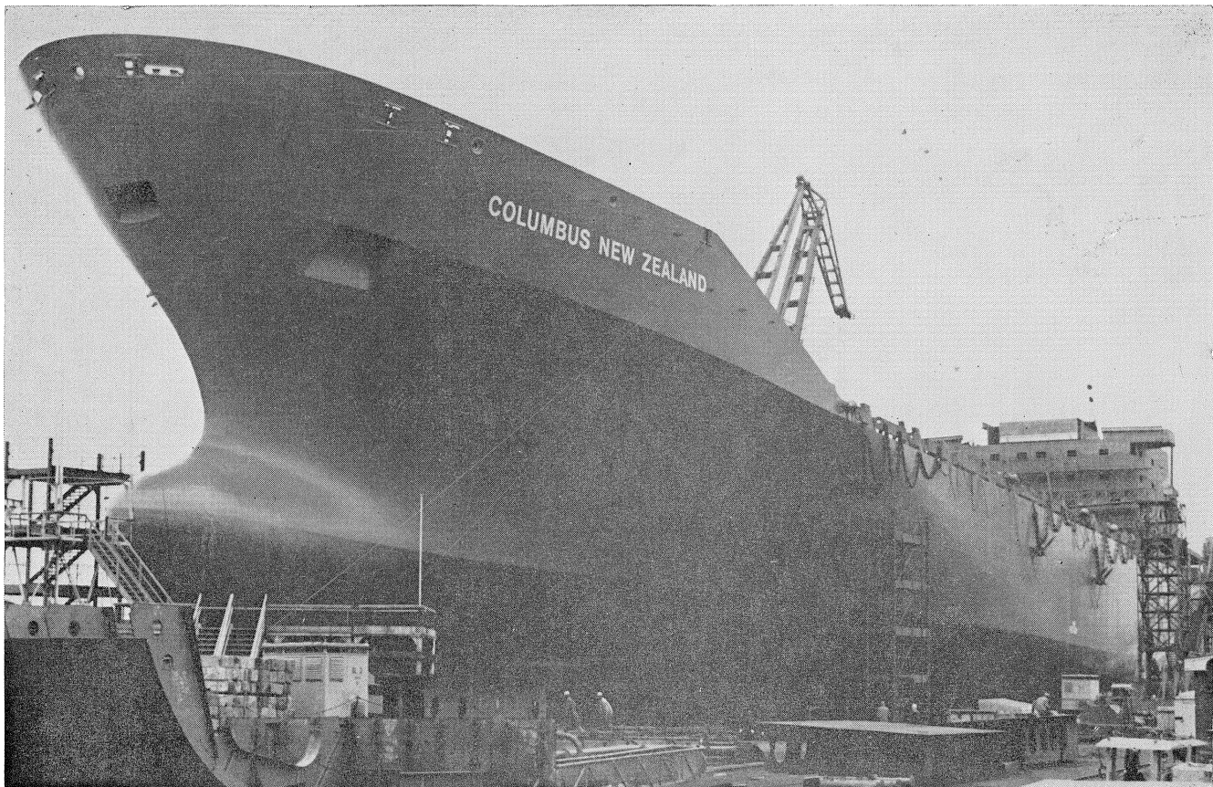
Cellular container ship Columbus New Zealand on the stocks at Hamburg. The distinctive bow construction is an aid to speed.
