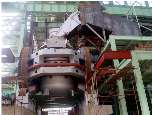
JCC Guixi (China): Cu scrap, internal material (slags), residues
