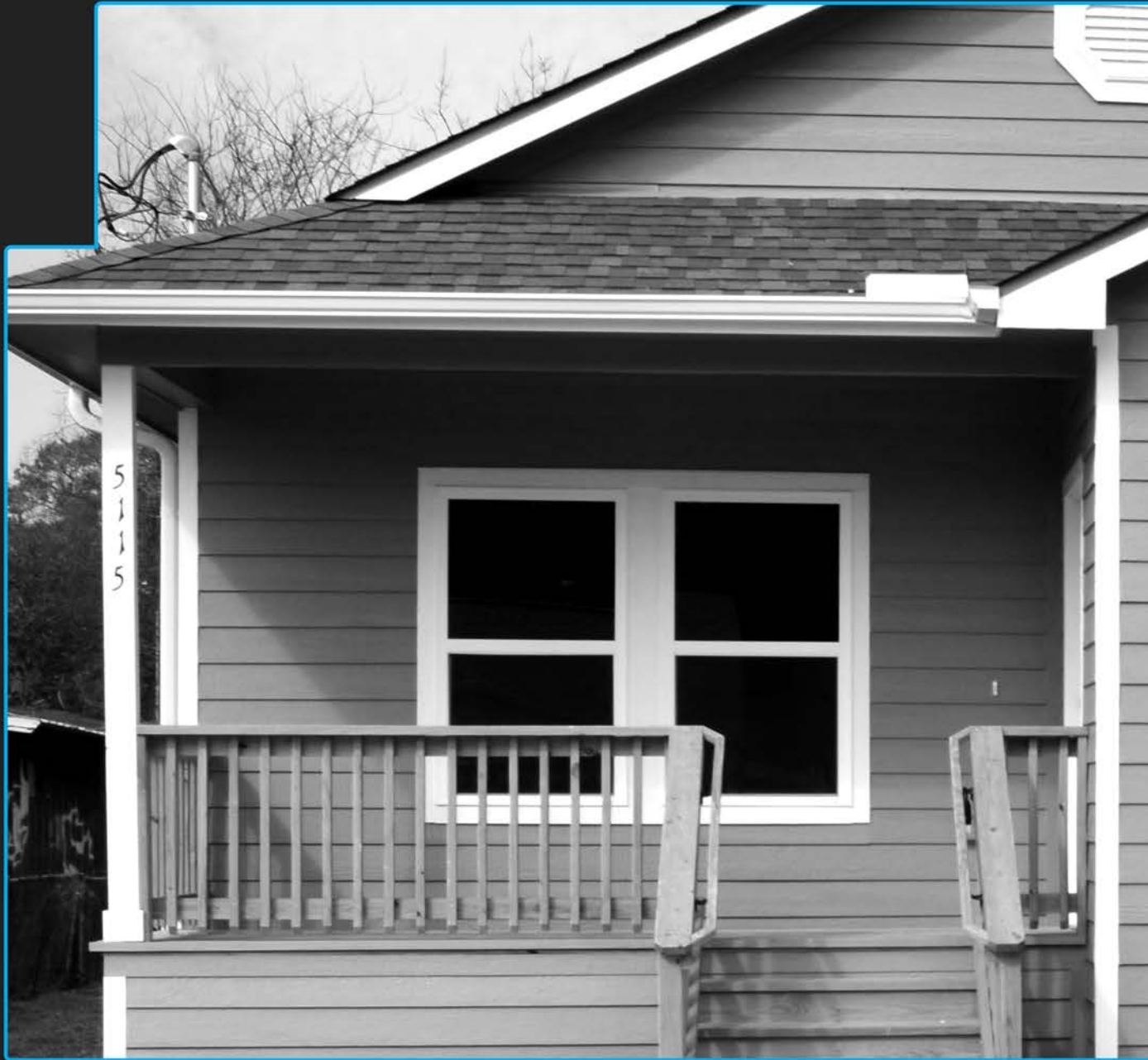
The Gutierrez family's newly reconstructed home - northside - District H | 3.3.2022 | Home Repair Program
