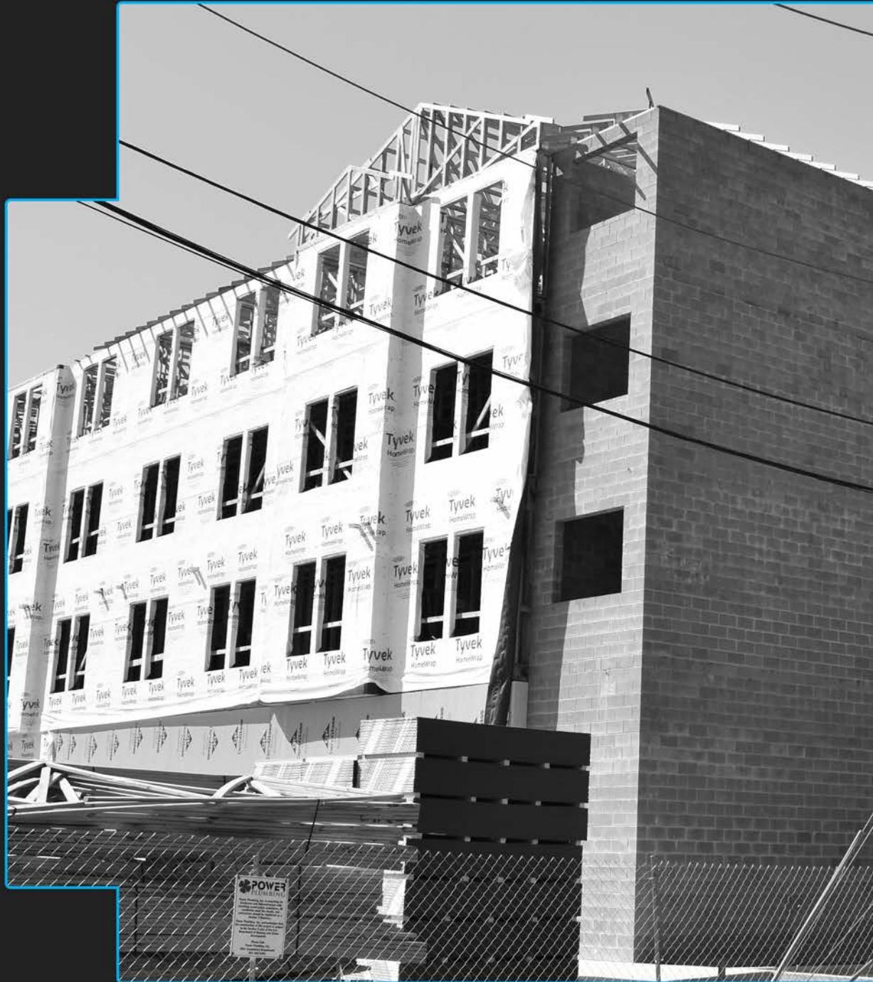
Harmony House | Multifamily | Groundbreaking | TIRZ, BONDS | Downtown Houston | 11.16.21
