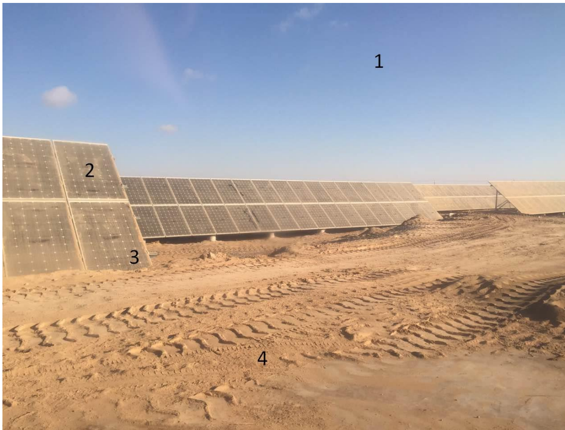
Fig. 32: Factors influencing dust soiling of PV modules in desert regions: 1 Climatic impact, ambient dust concentration, 2 Glazing characteristics, adhesion effects, non-uniform soiling, 3-Installation conditions, 4-Surrounding environment, dust particle characteristics. Photo: TÜV Rheinland Group
