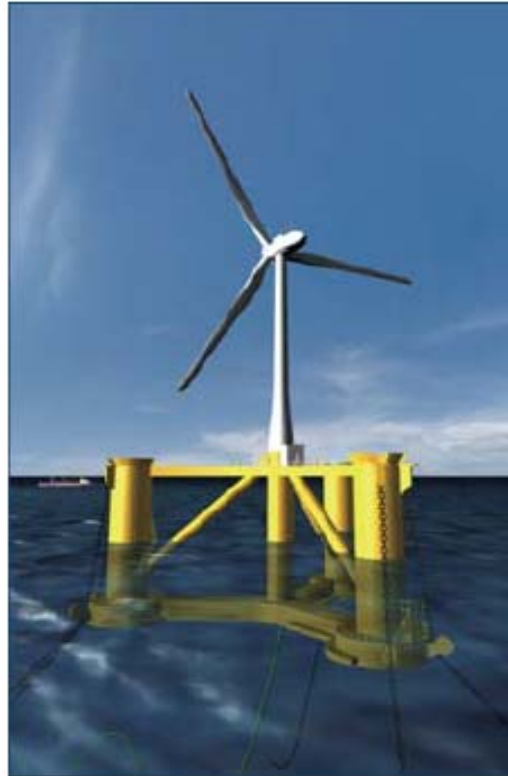
Compact Semi-Sub (2MW)
