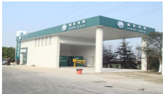
Charging/battery swap station in Baiyanghu Service area
