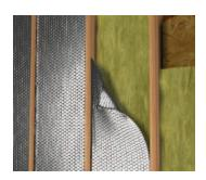
4. Wall - 2"x 4" R-14.0 Total Assembly (R-3.9 and a Vapor Moisture Barrier for the Reflectix®)
