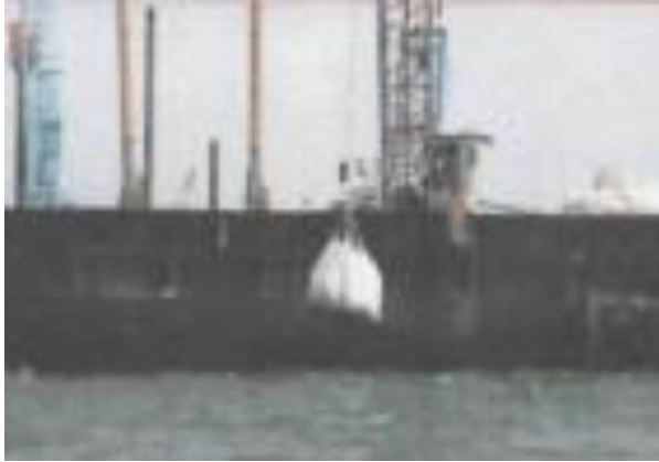
(5) buoy and concrete ballast placement
