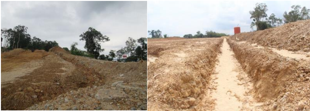
Figure 2.23 Drainage surrounding location.
