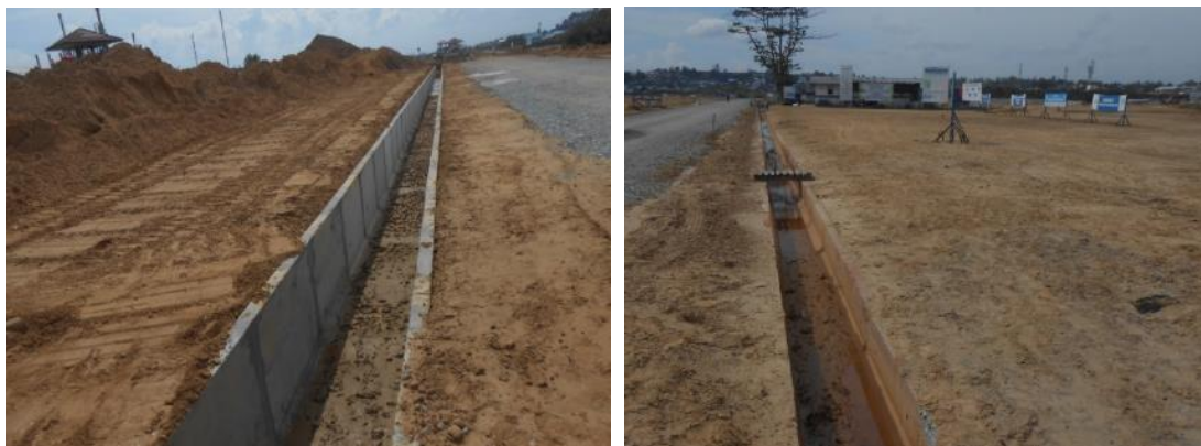
Figure 2.22 Run-off control ditches installed in construction and dumping areas.
