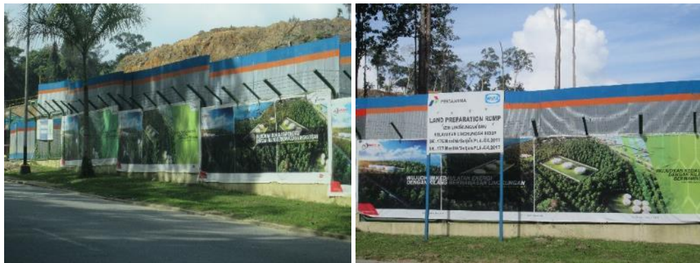
Figure 2.21 Fencing installed around the land clearing area.
