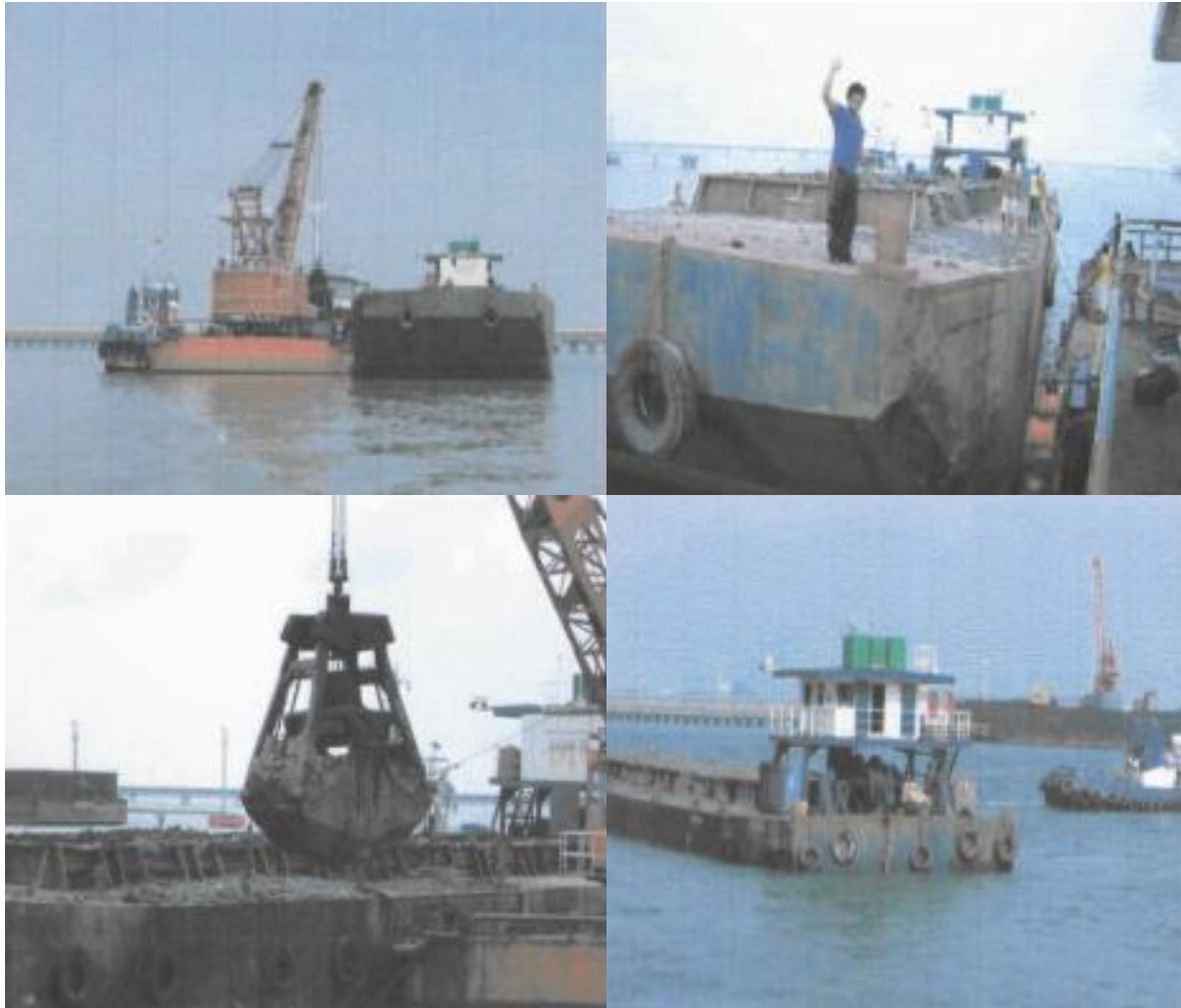
Figure 2.9 Illustration of dredging activity with clamshell method.
