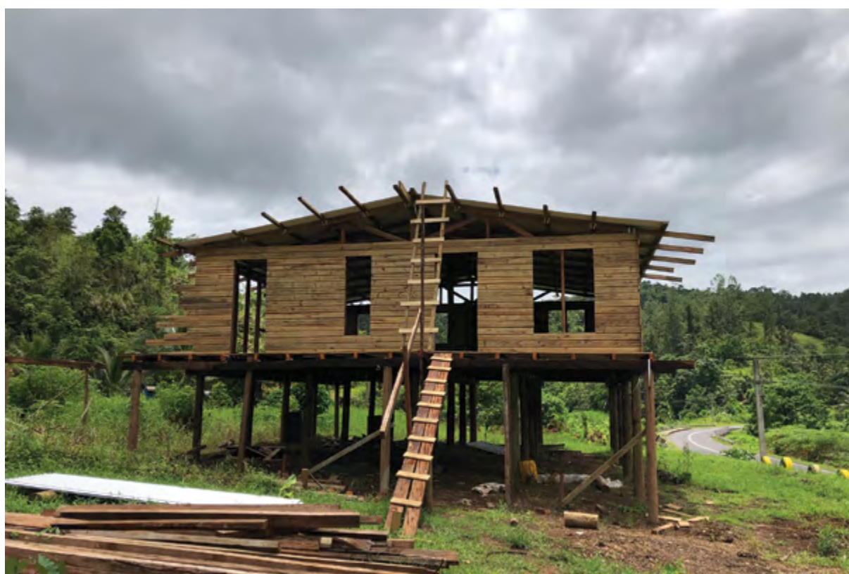
Building assessments in Fiji. Photo: Cyclone Testing Station, JCU.
