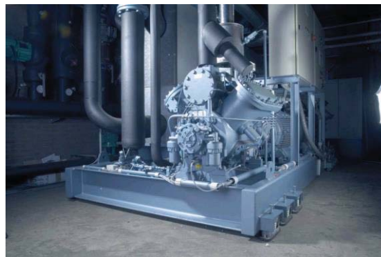
Figure 10-8: Typical KODI heat pump in Greenhouse
