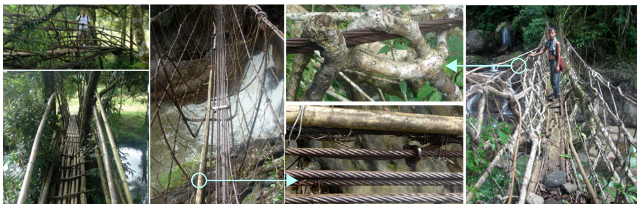
Figure 9. Bamboo bridge failure Figure 10. Steel suspension bridge failure Figure 11. Ficus-steel twining
