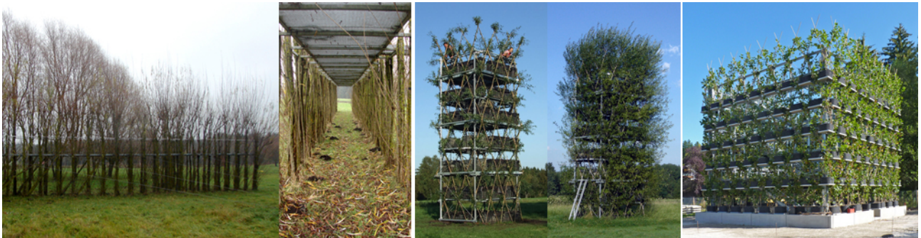
Figure 7. Footbridge (Ludwig F. and Storz O., 2005); Tower in the first and second year of development (Ludwig F. and Hackenbracht C., 2009); Plane Tree Cube Nagold (ludwig.schoenle, 2011)
