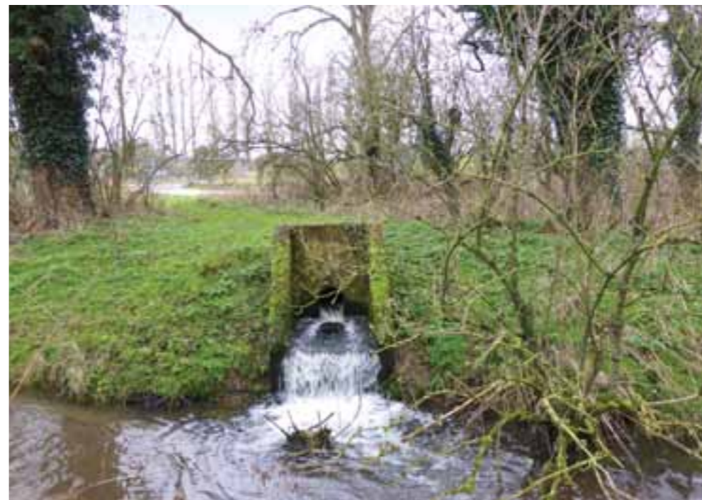
Photo 4. Outfall of Ingoldisthorpe Sewage Treatment Works.
