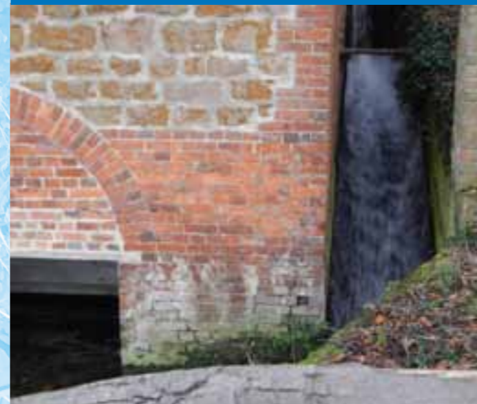
Photo 11. Main path of water through Snettisham Watermill.
