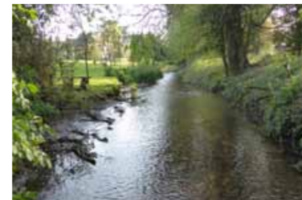
Before project – eroding banks
