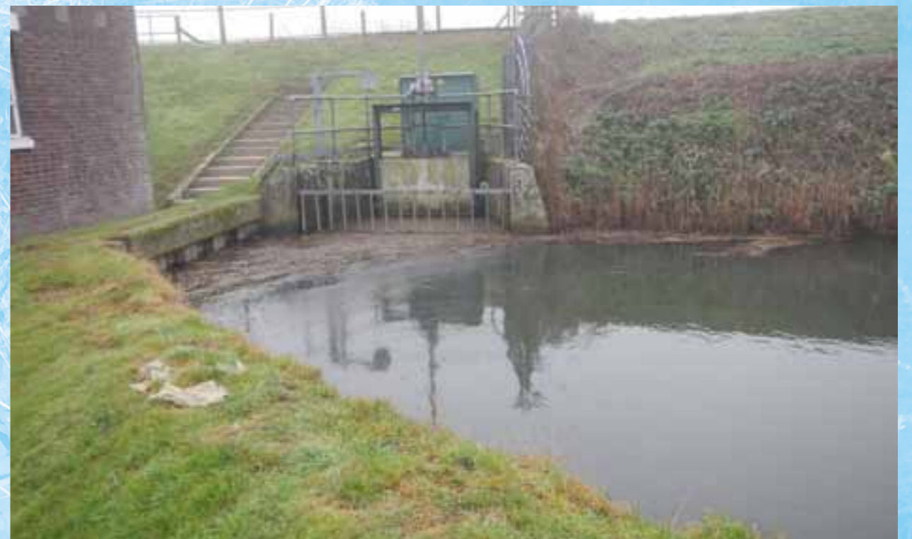
Photo 18. Sluice at tidal outlet.
