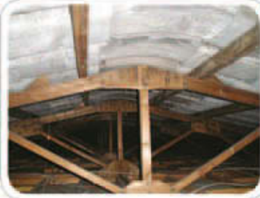
Greshams Pavilion Roof STABILISED
