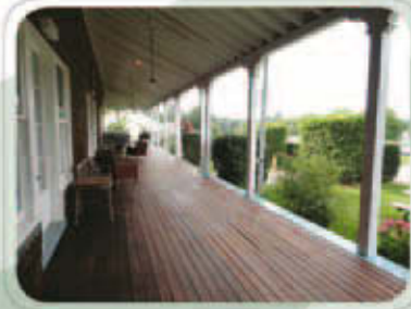
Canadian Pavilion Veranda STRUCTURAL REPAIR
