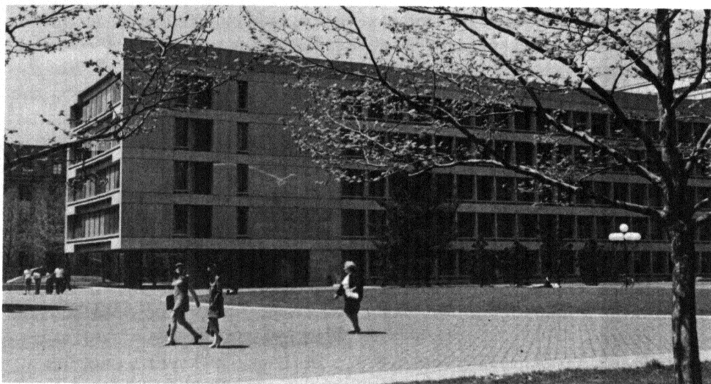
Dreyfus Chemistry Building at Massachusetts Institute of Technology. (Photo MIT)
