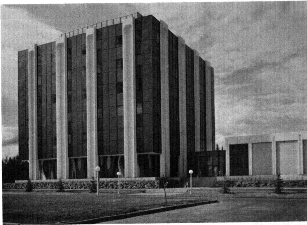
C. T. Elvey Building, The Geophysical Institute, University of Alaska. (Photo University of Alaska)
