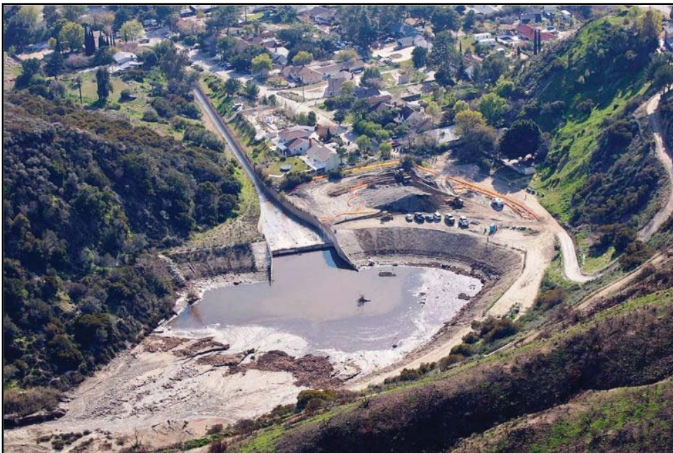
Figure 10.13: This debris basin in Los Angeles county is designed to capture the sediment, boulders, and other debris washed from the canyon during a storm.
