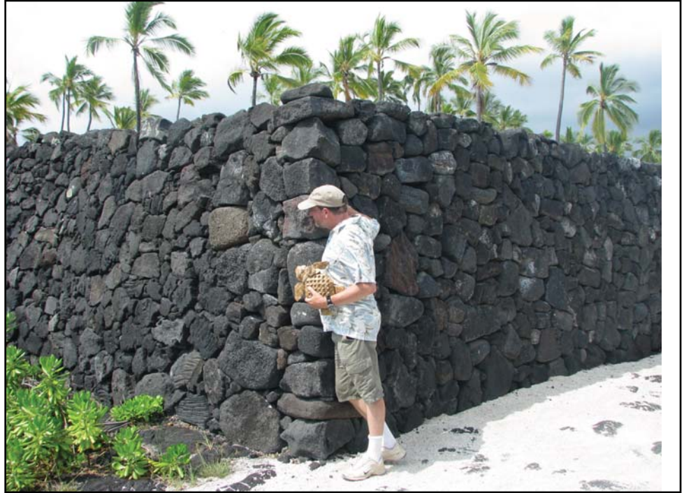
Figure 5.21: Impressive ancient dry stone construction at Pu'uhonua O Hōnaunau National Historical Park, Hawai'i Island.
