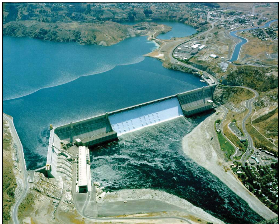
Figure 7.3: The Grand Coulee Dam.
