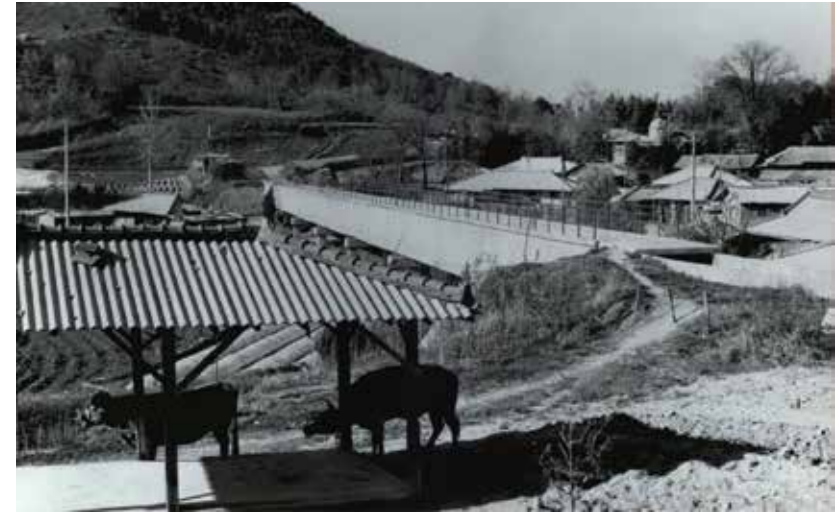
An irrigation network brought vital agricultural water to the farmers.
