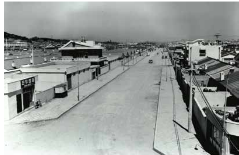
Modern housing built near industrial areas in Gwangju, Korea
