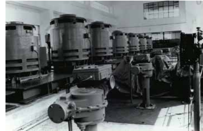
An irrigation network brought vital agricultural water to the farmers
