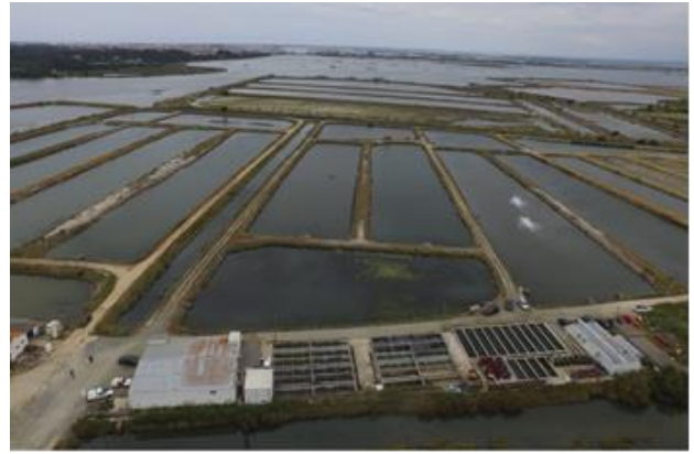
Figure 3: Integrated farm - fish ponds, macroalgae tanks and supporting buildings © ALGAplus, 2019 For reproduction or use of this material, permission must be sought directly from the copyright holder.
