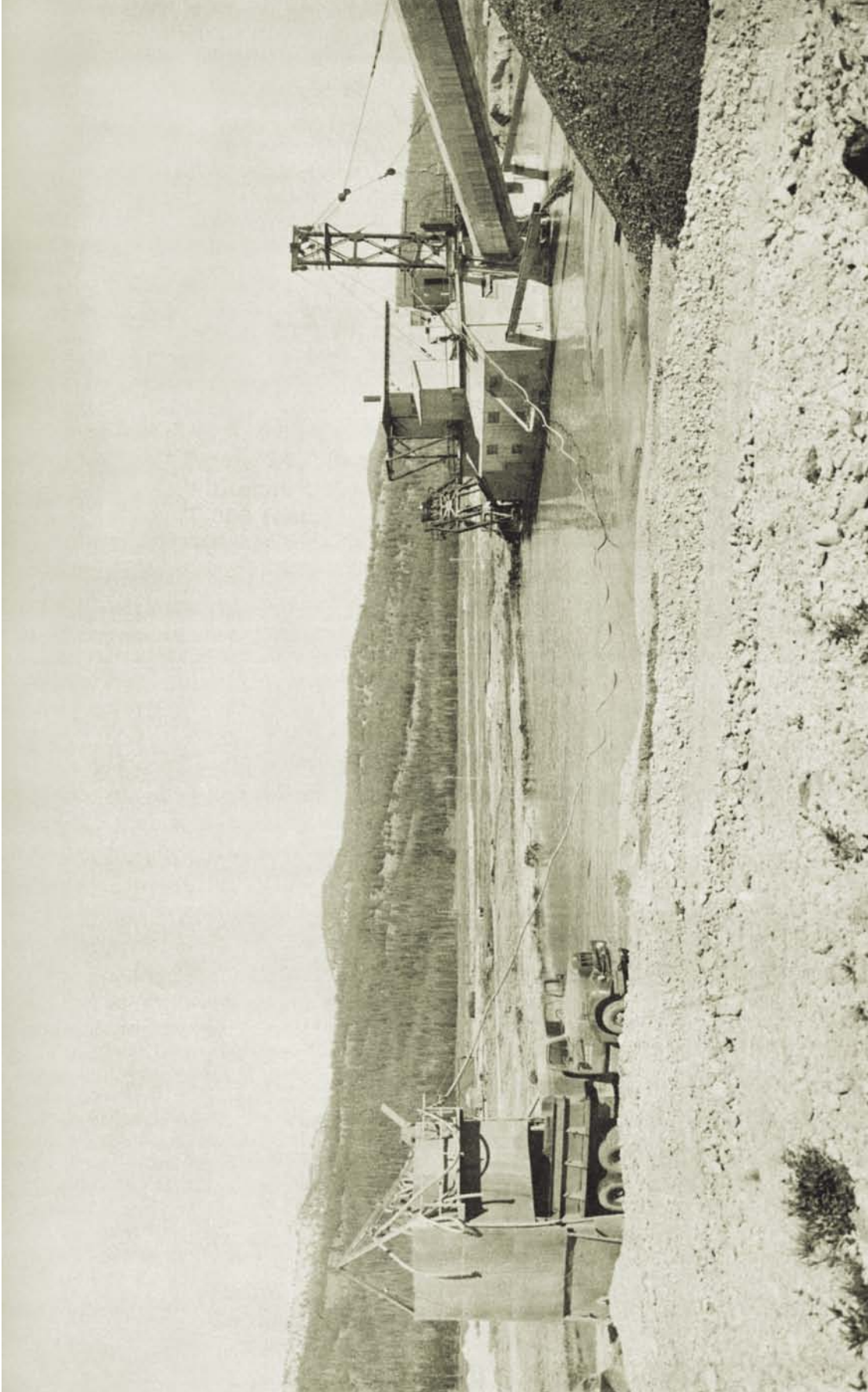
Figure 20. Porter Brothers dredge in Bear Valley, Idaho, worked columbium (now called niobium)-tantalum placer deposits. This dredge operated from 1955 to 1960; exact date of photograph is unknown. Monazite was produced as a byproduct from these placer deposits. (Photograph from Savage (1961, fig. 13); used with permission of Idaho Geological Survey.)
