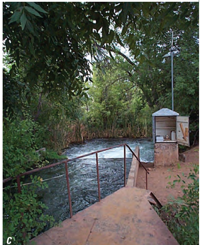
Figure 13. A–C, Instrument shelter located on a dam.
