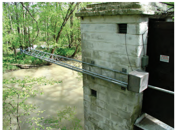
Figure 19. Cantilevered wire-weight gage.
