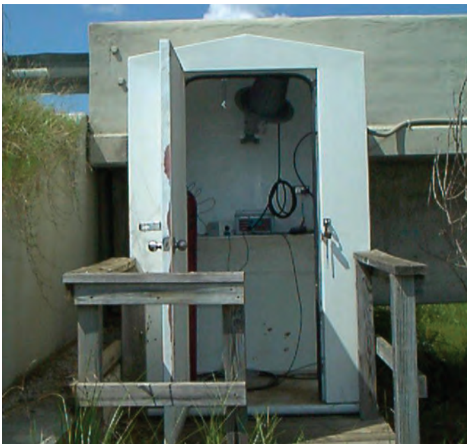
Figure 12. Instrument shelter located on a bridge abutment.
