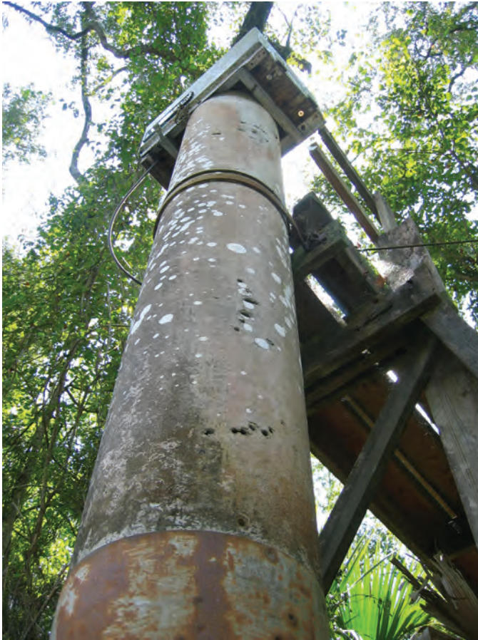
Figure 3. Concrete pipe stilling well and shelter.
