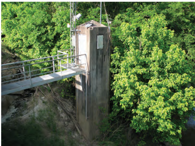
Figure 1. Reinforced concrete stilling well and shelter.
