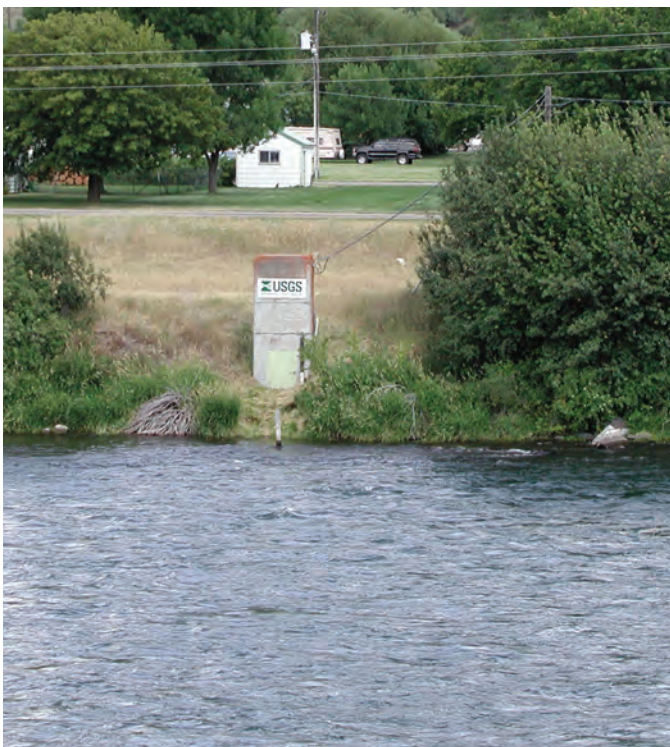
Figure 4. Concrete block stilling well and shelter.
