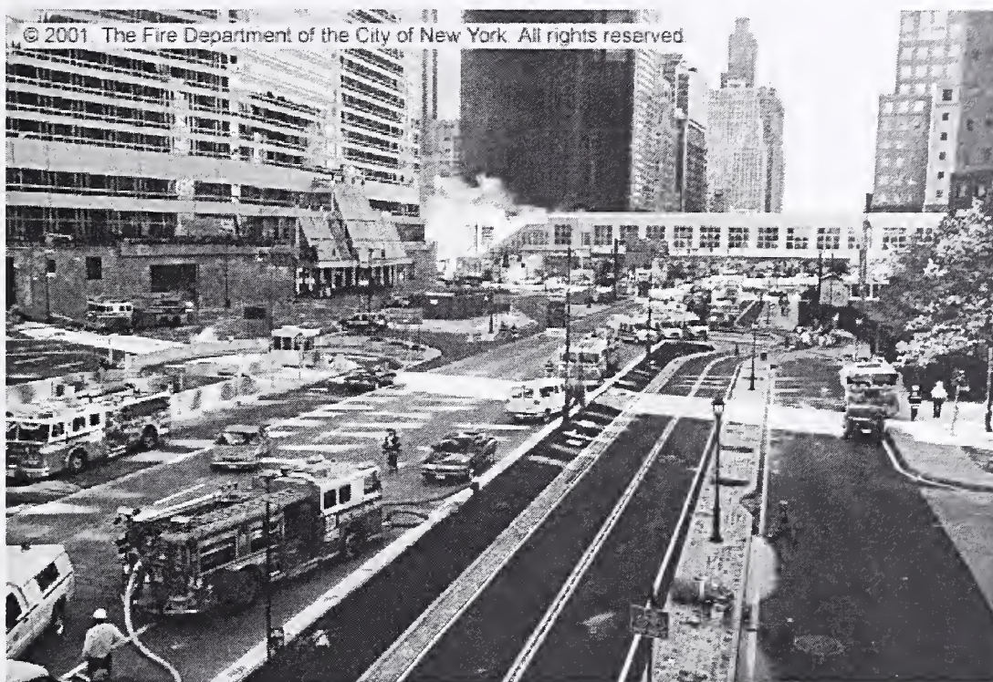
Figure 5–14. Photograph taken from near the corners of West and Vesey Streets looking south before the collapse of WTC 2.
