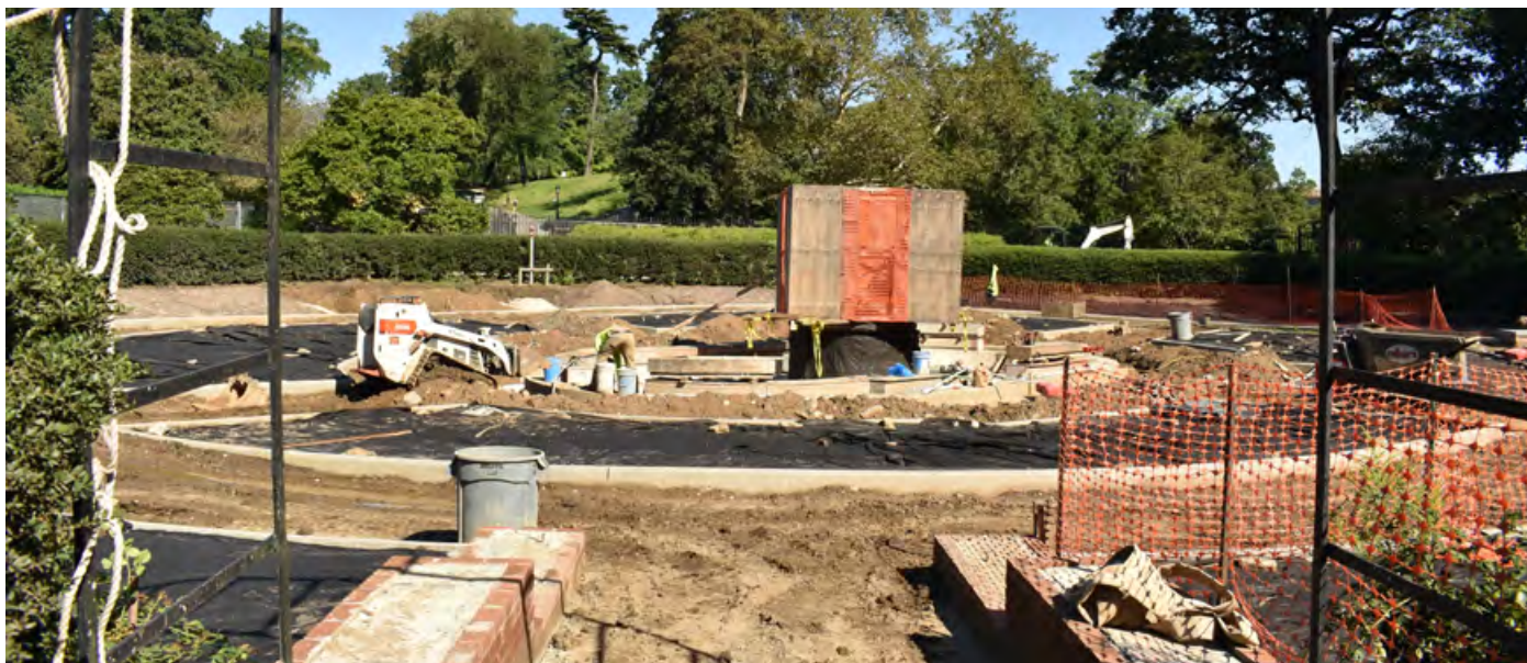
Fountain and drainage work in the French Garden
