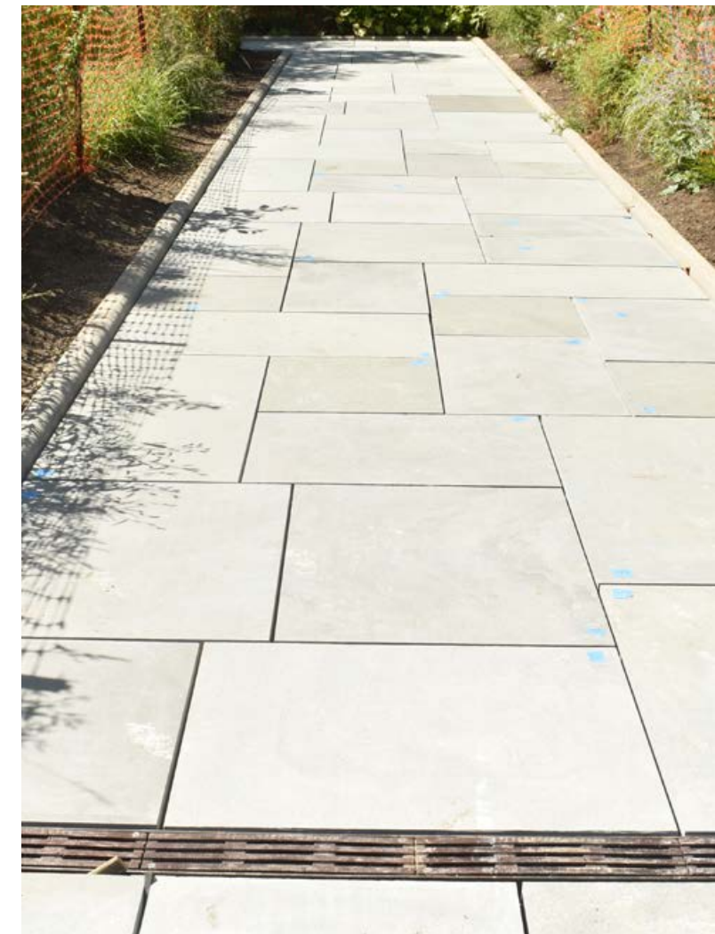
A completed pathway
