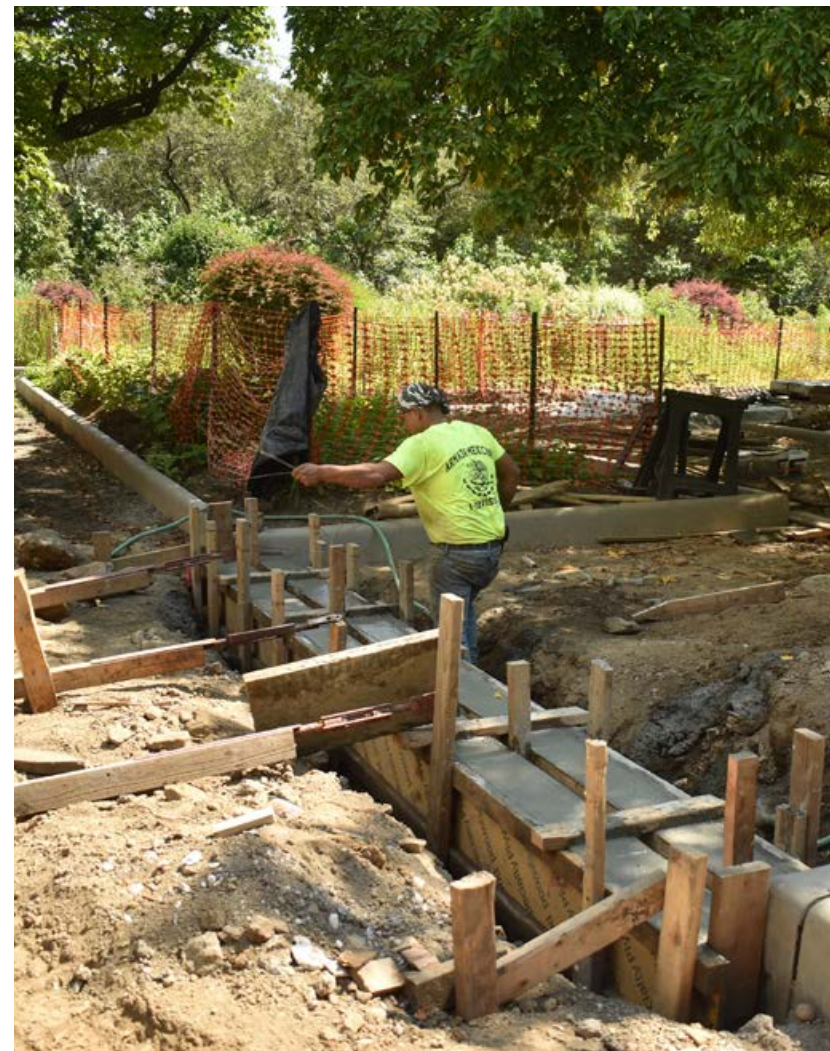
Irrigation work in the South Garden
