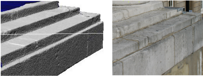
Figure 2: Comparison between a laser scanning model (left) and an image taken from a similar viewport (right). © Moysiadis, University College London
