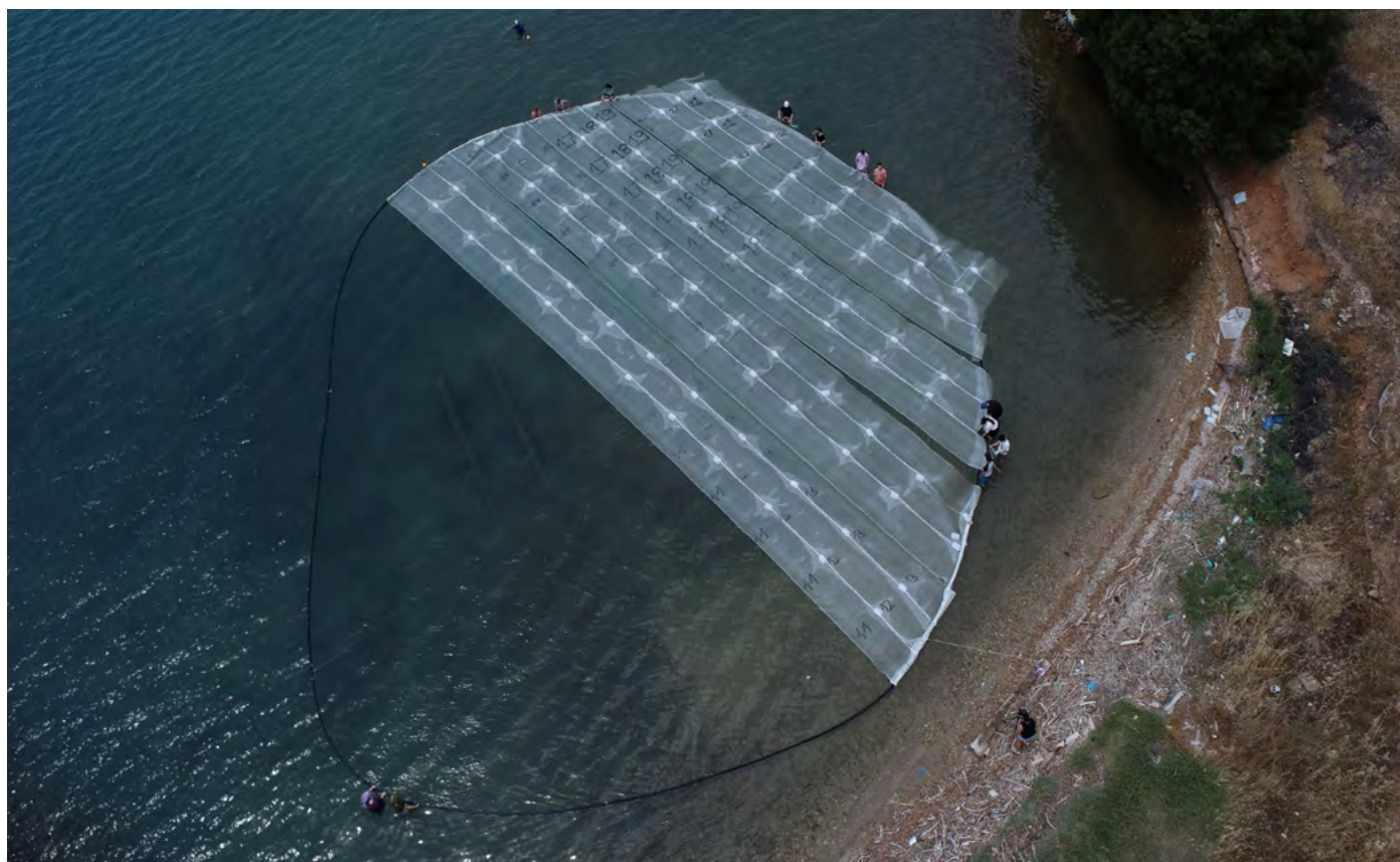
Figure 1. HDPE 28 m diameter target during construction showing the white HDPE mesh sheets.
