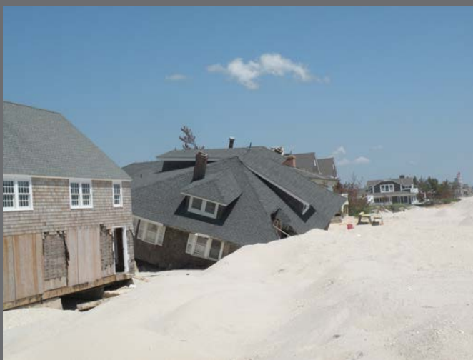
Beach houses in New Jersey were destroyed by Hurricane Sandy.
