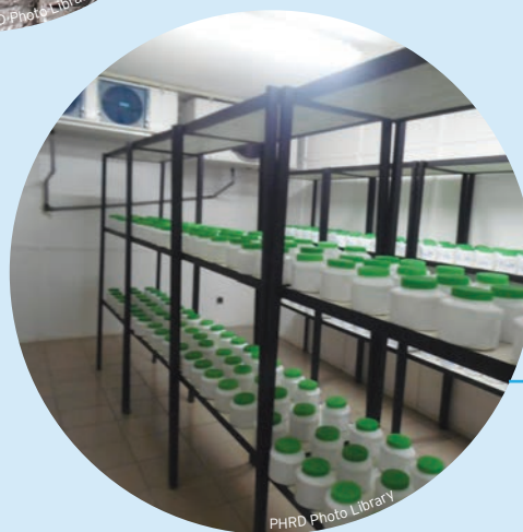
Inside View of the Rice Seed Storage Cold Room in Côte d'Ivoire
