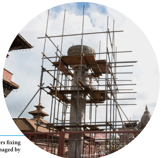
Before: Damaged building during earthquake
