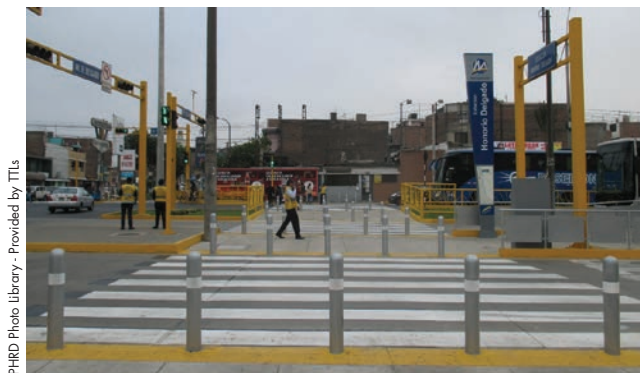
Peru - PHRD grant funded a pedestrian traffic island level with the vehicular lanes in the surroundings of the Honorio Delgado Station.
