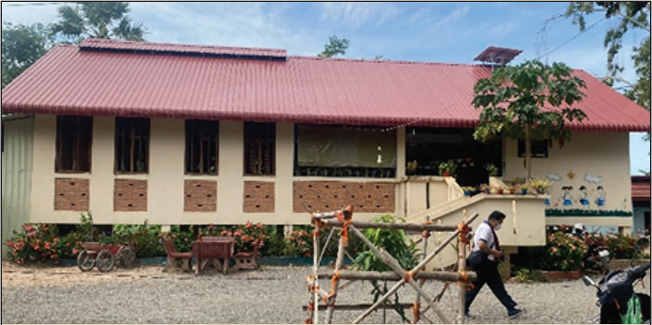
A project in Cambodia included activities such as constructing floating and onshore centers that provide enabling environments for better learning outcomes for children.
