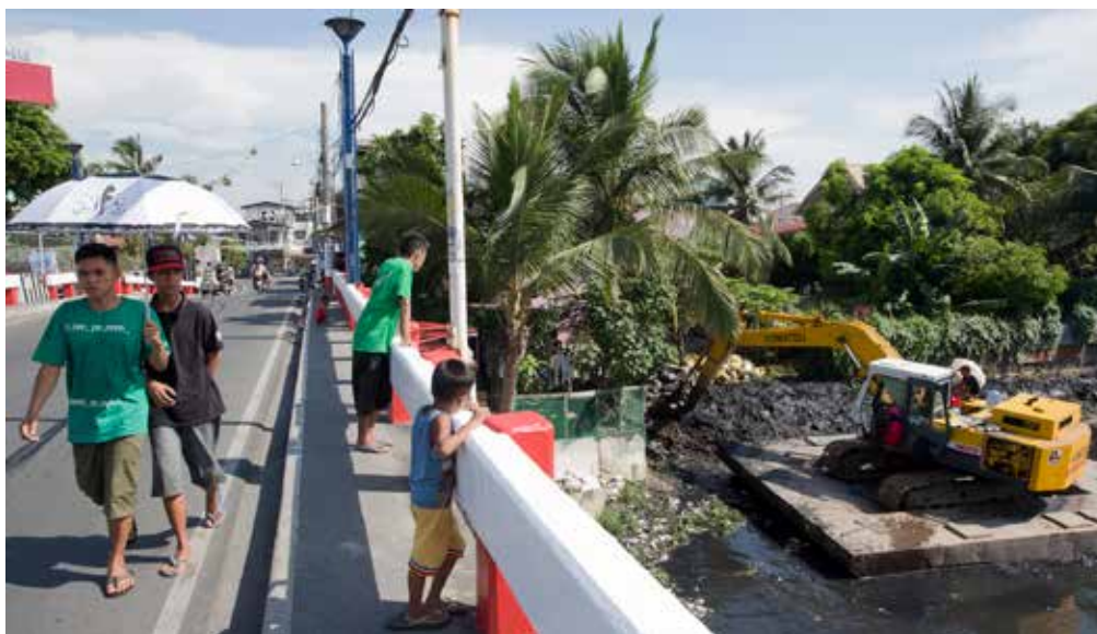
Pedestrians watch as city workers dredge the riverbed of the Taguig River, Philippines. Photo: Dominic Chavez/World Bank.
