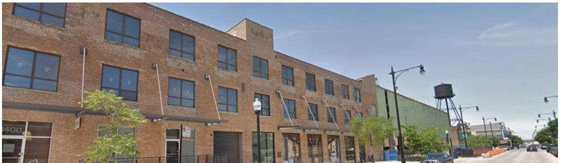
Industrial/Office buildings on the Southern side of Kingston Street, consistent with the Zoning map in the plan Source: © Google Maps, Intersection of Weed and N Kingston Streets, https://tinyurl.com/ycfw7a2j
