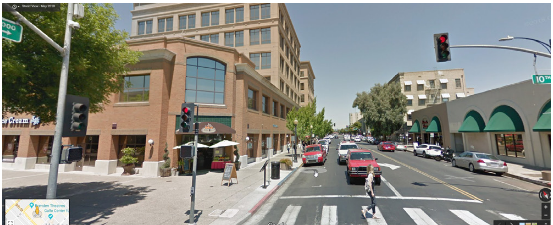
This is the street image of 1010 10th Street Building and J Street (Facing north). Source: © Google Maps https://www.google.com/maps/@37.6405427,-121.0002471,3a,75y,16.78h,83.44t/data=!3m6!1e1!3m4!1sHoNjz55acA6NpD2qcES08A!2e0!7i13312!8i6656
