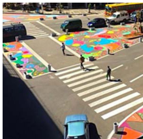
Figure 7. Addis Ababa reduced lane widths and turning radii for motor vehicles in order to improve pedestrian safety. (Images: NACTO/Global Designing Cities Initiative)
