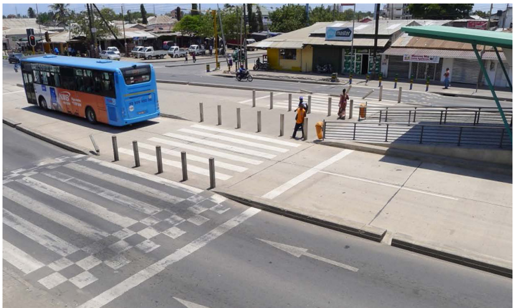
Figure 5. Raised zebra crossing, a traffic calming measure, contributing to a safe walking and cycling environment in Dar es Salaam.
