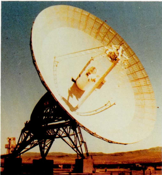
The 64-meter radar telescope of the JPL Goldstone Tracking Station in California's Mohave Desert. Normally used for tracking and communication with spacecraft, this facility can also be operated as a radio or a radar telescope. Richard Goldstein and his colleagues used this telescope in 1973 to make the first radar detection of Saturn's rings, which proved to be remarkably efficient reflectors of microwaves.
