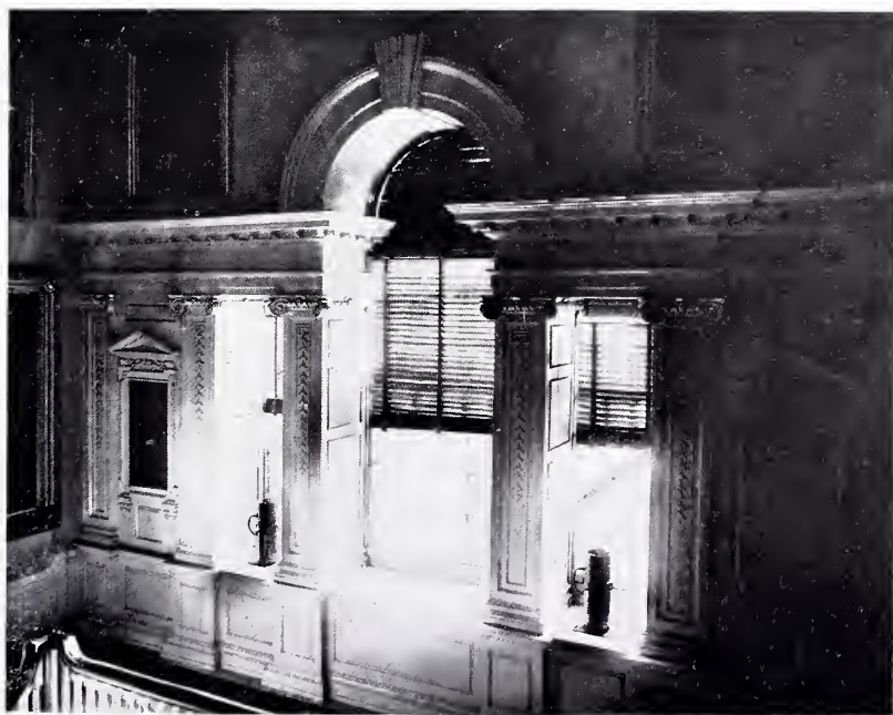
PLATE LXXVIII. — Stairway Landing, Independence Hall; Palladian Window at Stairway Landing.
