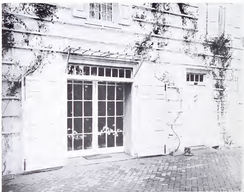
PLATE XIII. — Wyck, Germantown Avenue and Walnut Lane, Germantown. Erected by Hans Millan about 1690; Hall and Entrance Doorways, Wyck.
