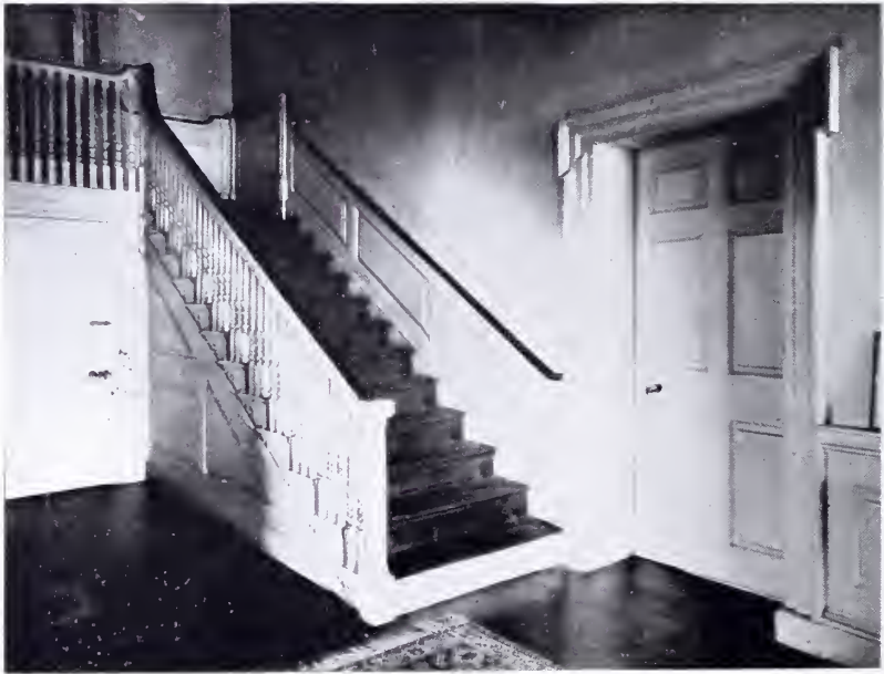
PLATE LVII. — Hall and Staircase, Cliveden; Staircase Detail, Cliveden.
