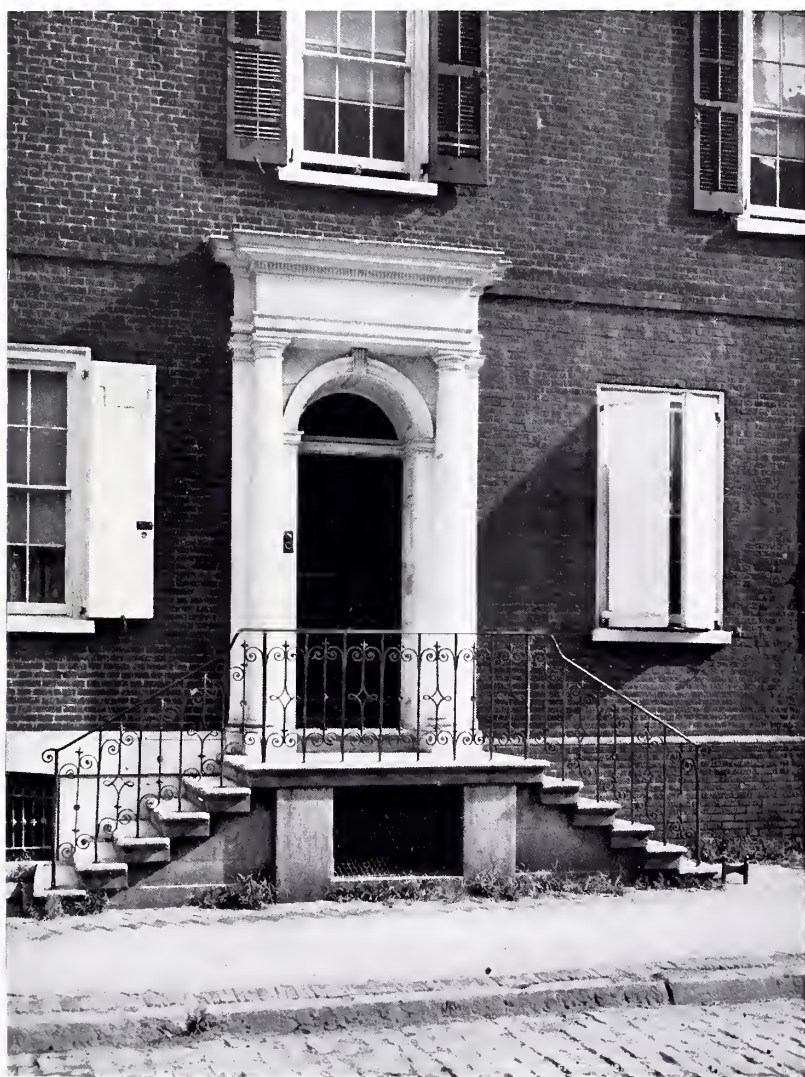
PLATE XXVIII. — Doorway, 301 South Seventh Street.
