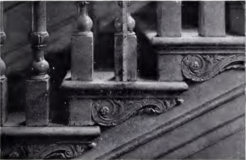
PLATE LX. — Detail of Stair Ends, Carpenter House, Third and Spruce Streets; Detail of Stair Ends, Independence Hall (horizontal section).
