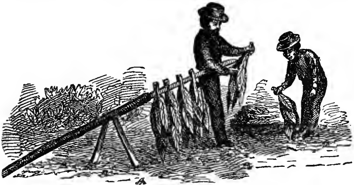
PUTTING ON LATH.
