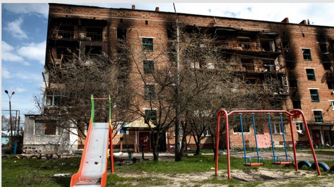
Apartment building in Ukraine which suffered the attack of Russian armed forces. Photo: Freepik
