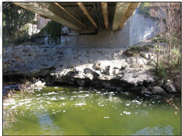
Bank Protection under bridge at CTP
