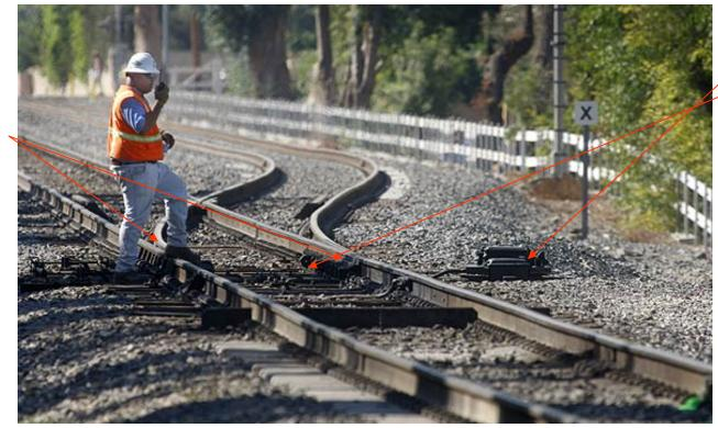
Switch Box and bars that were destroyed When the train "ran through" The Switch
