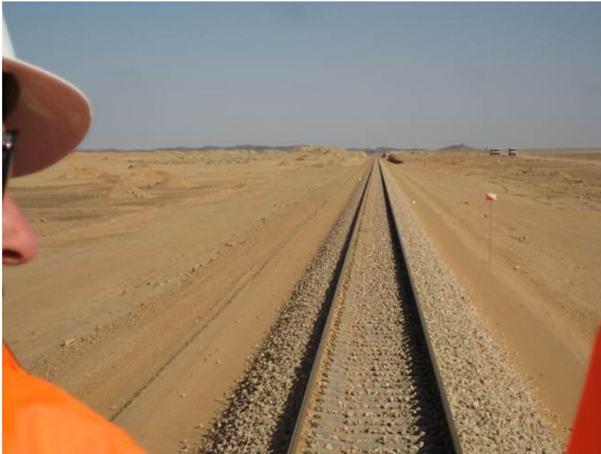
1. Single Track with provision for dual track
