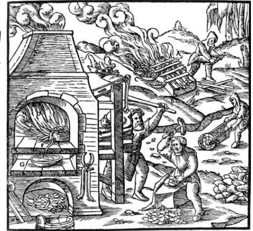
A—WOOD. B—BRICKS. C—PANS. D—FURNACE. E—CRUCIBLE. F—PIPE. G—DIPPING-POT.
