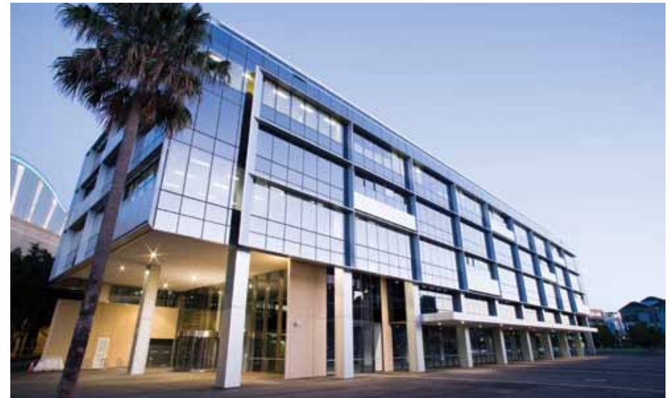
workplace 6 , Sydney, 6 Star Green Star – Office Design v2, 6 Star Green Star – Office Design As Built v2
