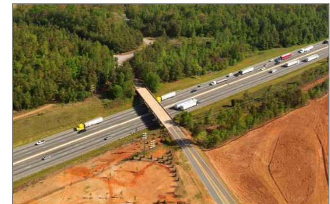
Salters Road/Old Sulphur Springs Road Overpass
