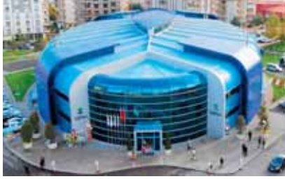
The Alleben 1 swimming pool is located in Şehitkamil district of Gaziantep province.
