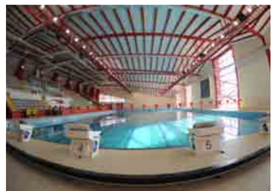
Olympic Swimming Pool
