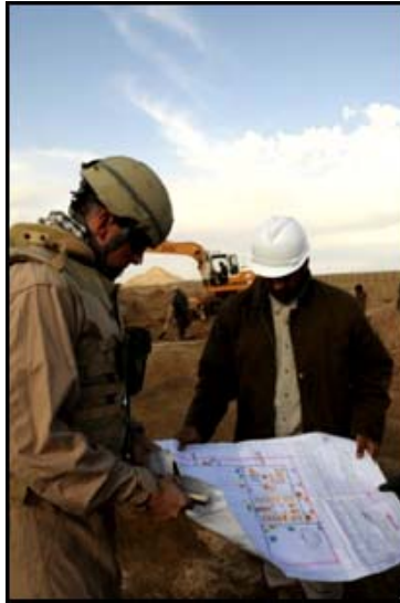
Afghanistan construction project
