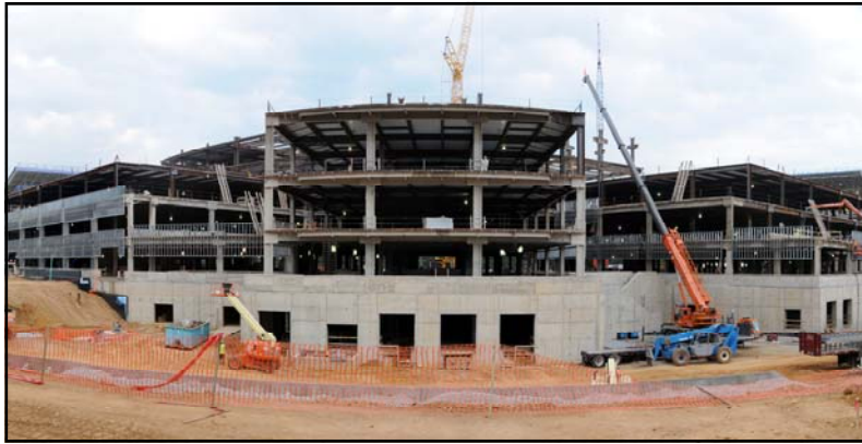
New hospital at Fort Belvoir, VA
