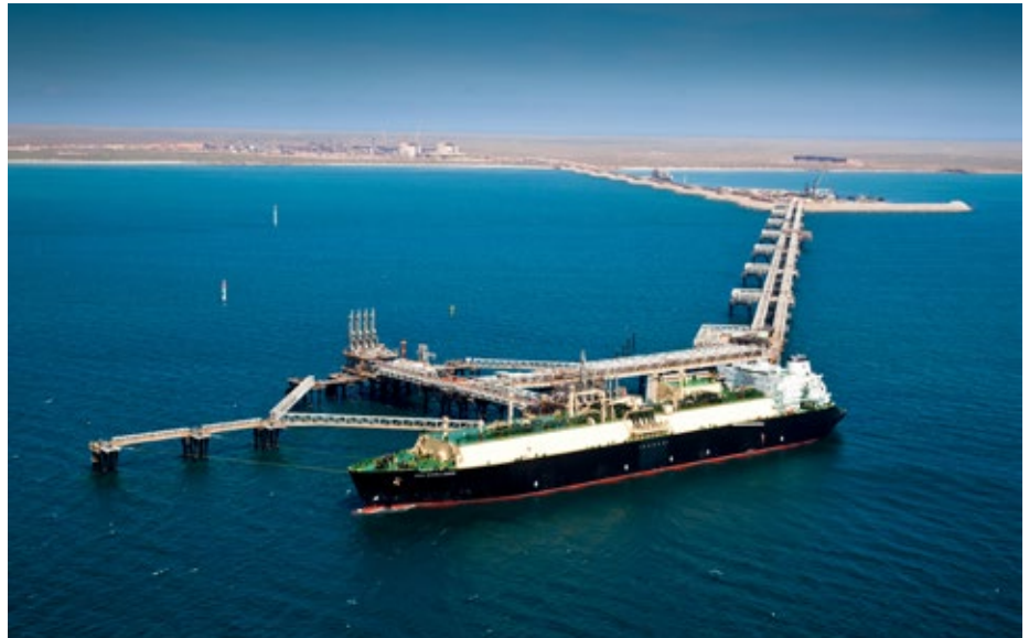
The Gorgon LNG plant in Australia. Its first train is now operating at 85% capacity. (Chevron)
