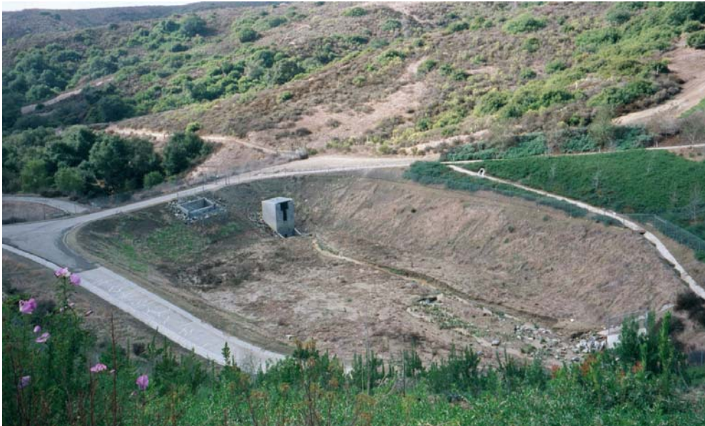
Figure 4: The Wood Canyon Creek at J02P08 – Pre-construction View
