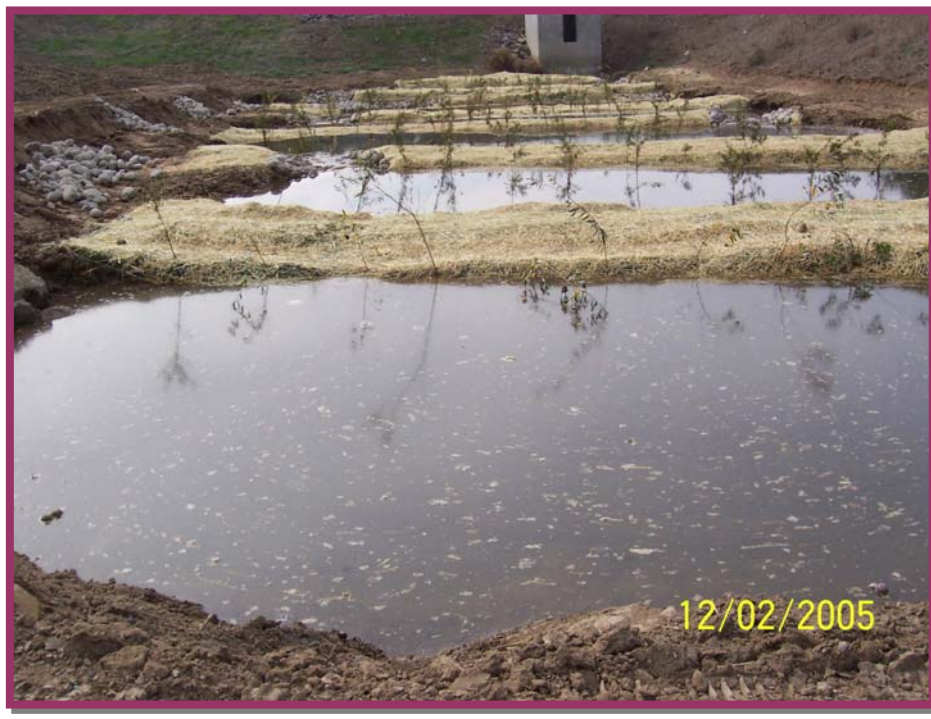
Figure 5: The Wood Canyon Creek at J02P08 – Post-construction View of the Ponds
